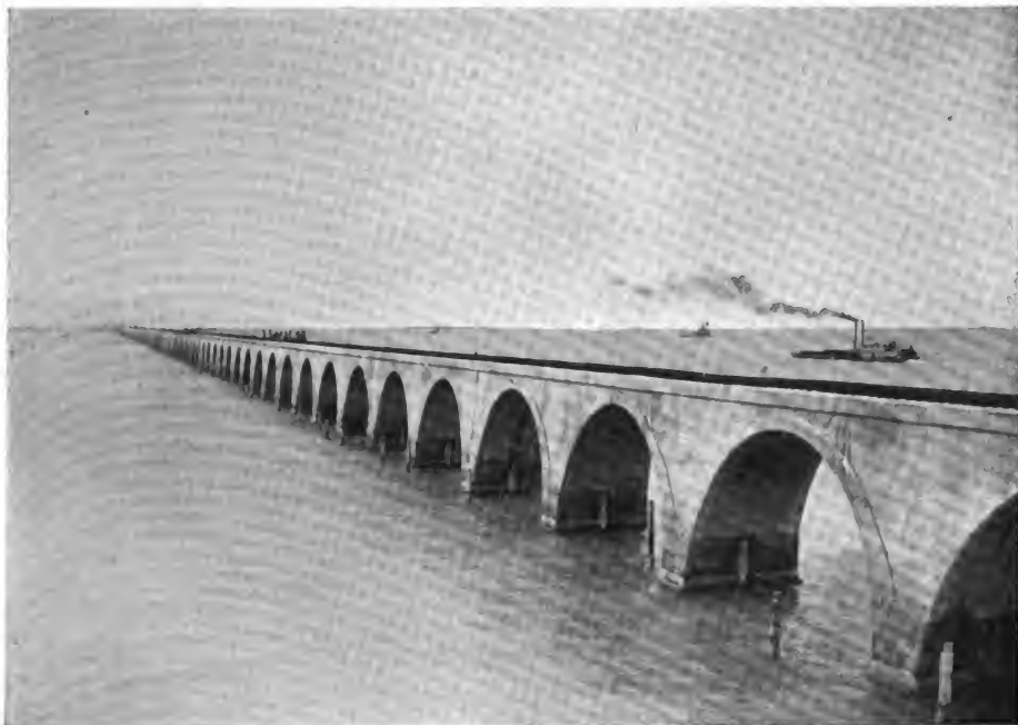
Long Key Viaduct. —Height of rails above tide level, 31 feet. In crossing the viaduct trains go practically out of sight of land.
